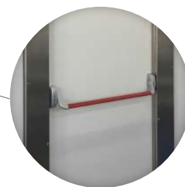
Fire Rated Panic Bar in the back of the door
