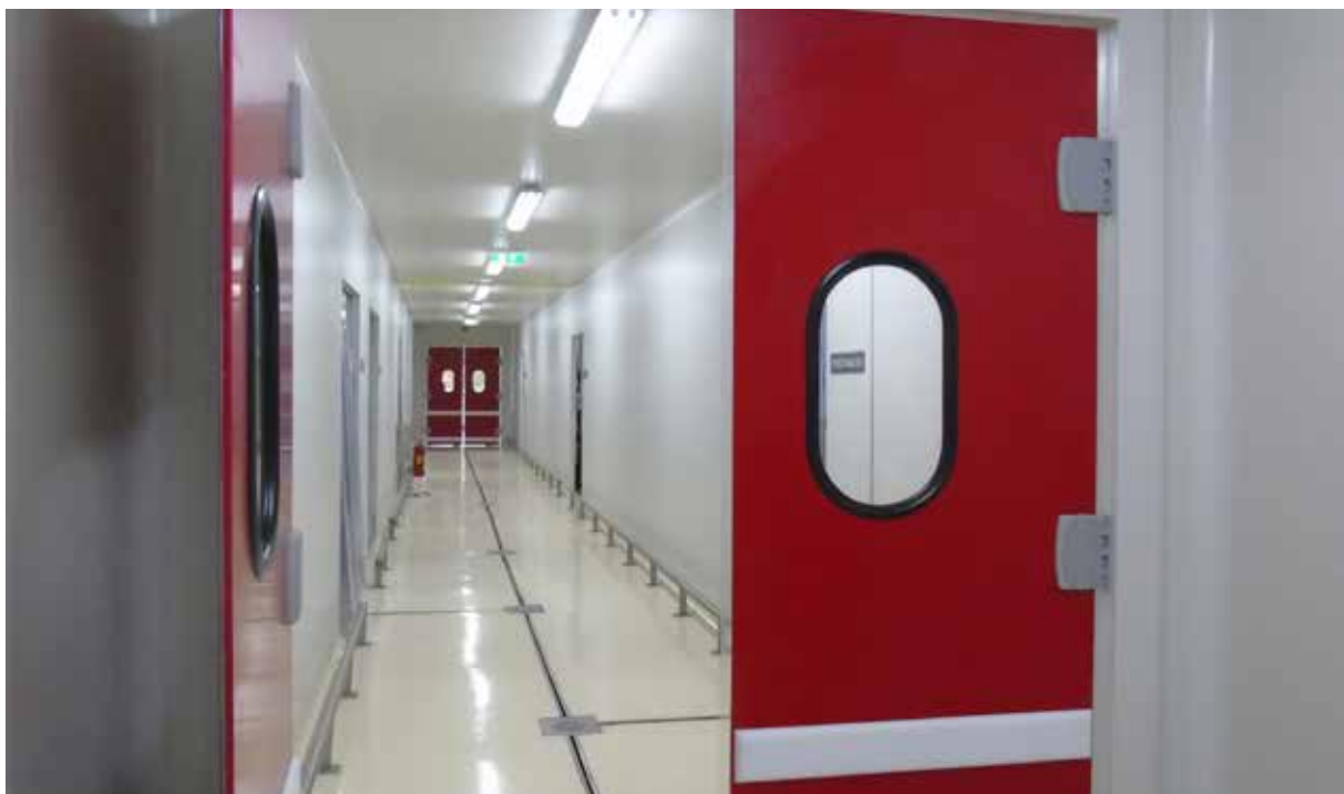
Hallway with swing polyethylene doors
