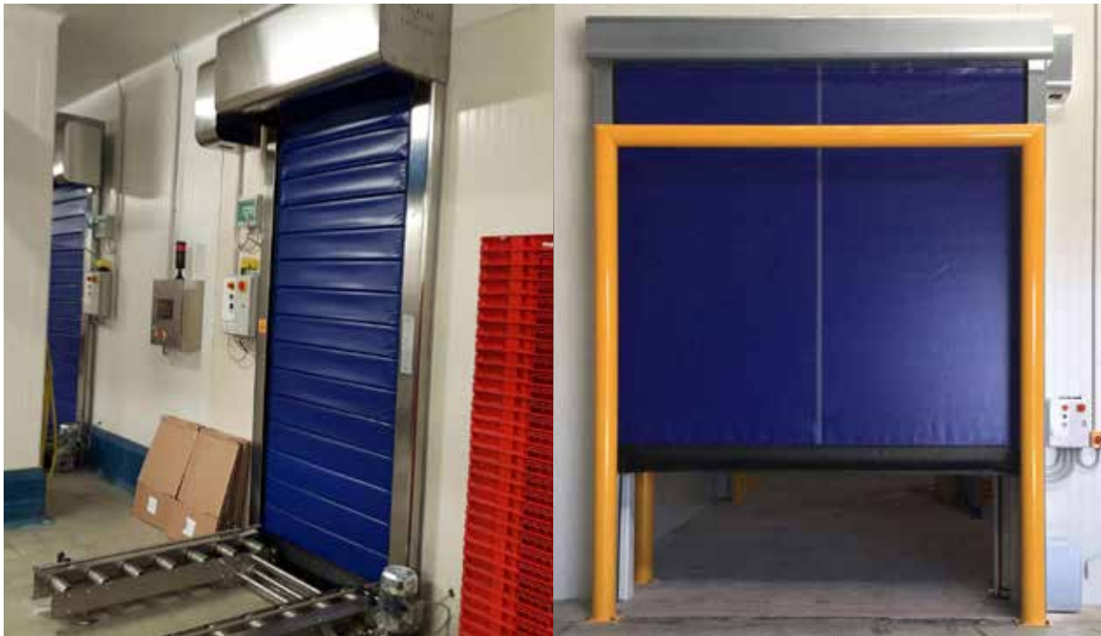
Cold storage fast roll doors on cold rooms
